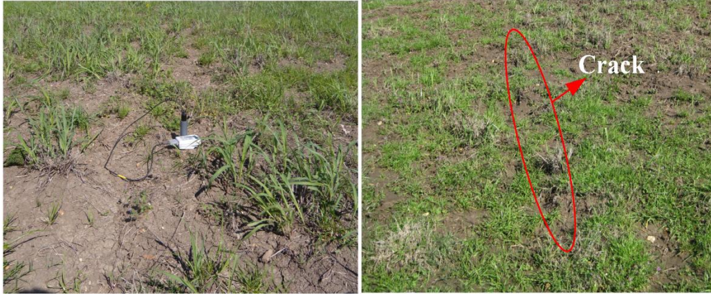
Figure 13 Sparse grass (left) and cracks (right) in FP2 observed after the UAVSAR image acquired for this study.
